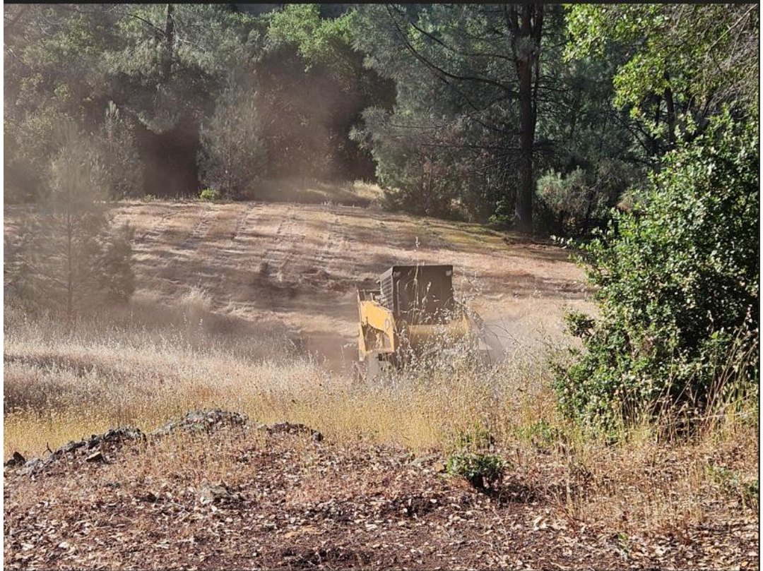
Mastication at Willow Creek Court
